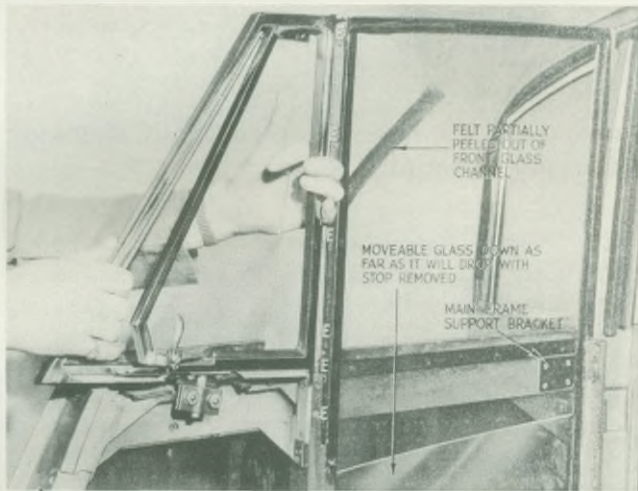
Fig. 20. The front vent light frame being removed from the door body
