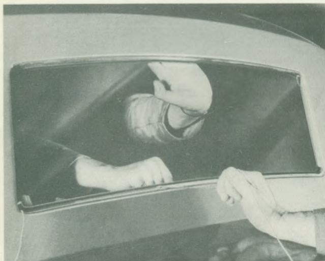
Fig. 32. The rear light being held firmly in position whilst the flanges of the glazing rubber are pulled out to lay along the aperture edges. A length of string laid around the rubber first can be used (as shown above) to assist in this operation.
