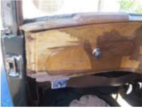
An extreme example of decay!
